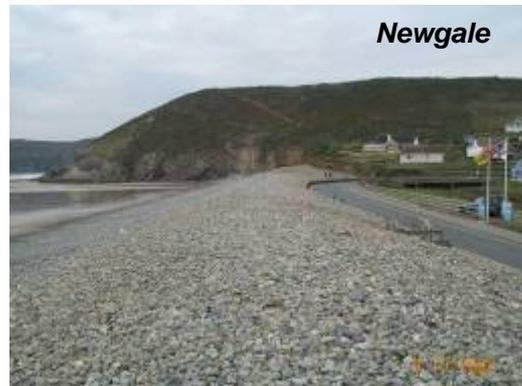
In the valley immediately behind the road there are several properties and a petrol station which have all been affected by flooding and the overtopping of shingle. The road is maintained by shingle clearance on a regular basis. The road crosses a bridge over the Brandy Brook and then rises up through the main part of the village, continuing well in land of the coast over the higher ground at the northern end of the Zone.
