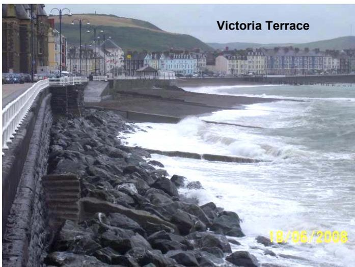
The frontage experiences overtopping and deposition of shingle on the promenade. The level of defence south of the Pier is around 9m AOD but, with only the exposed hard shoreline of Castle Rock, waves directly hit and overtop the promenade wall on a regular basis. The level of the promenade at Marine terrace is around 4m AOD and waves run up the shingle back slope to flood the promenade. At Victoria Terrace the defence level is around 6m AOD and
