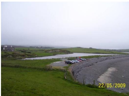
At the eastern end there may already be seen some increasing pressure on the defence. The shingle beach is lowering and this process is likely to continue with sea level rise. As the shingle bank, in general, moves back, so the end of the defence would be
